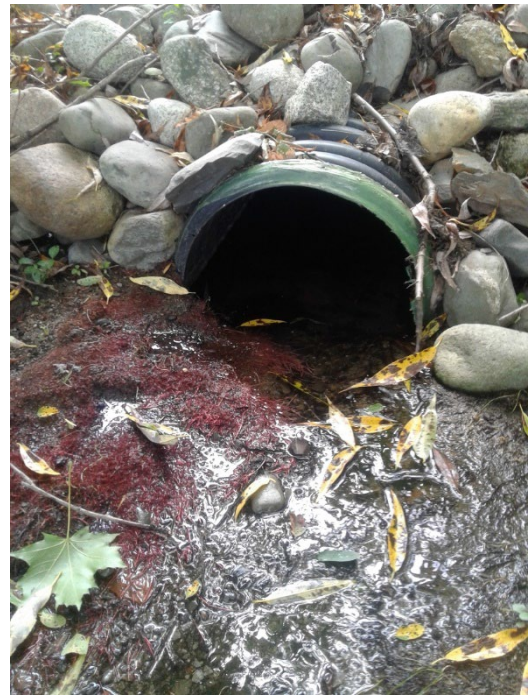
Fig. 2. This outfall is partially submerged and a clean catch of its discharge is not possible.
