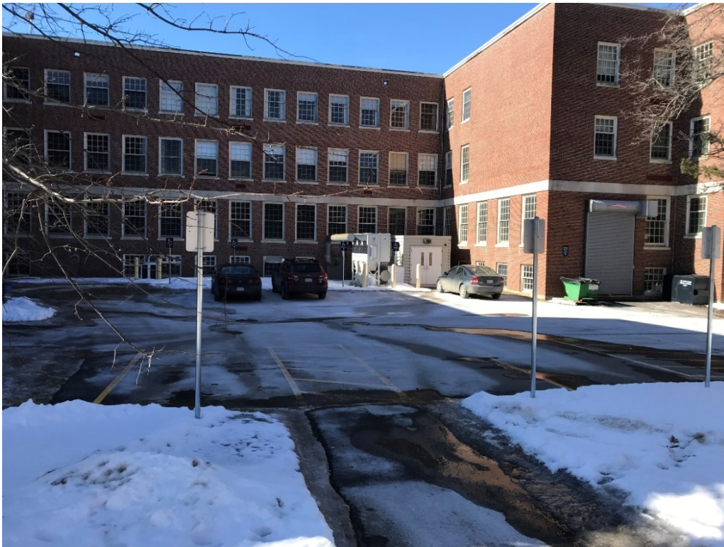
View of Boardman and Parking/Service Area from Sidewalk – Mid Way along MTL
