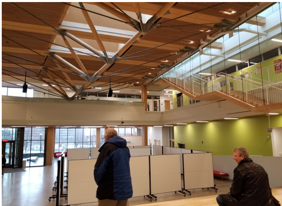
Commons – showing wood/steel truss system
