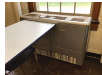
Bottom Right: A radiant heater cabinet in classroom 216, below the window
