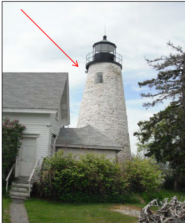
Photo 2-1. Dice Head Lighthouse, Castine, ME. Red arrow depicts location of paired detectors.
