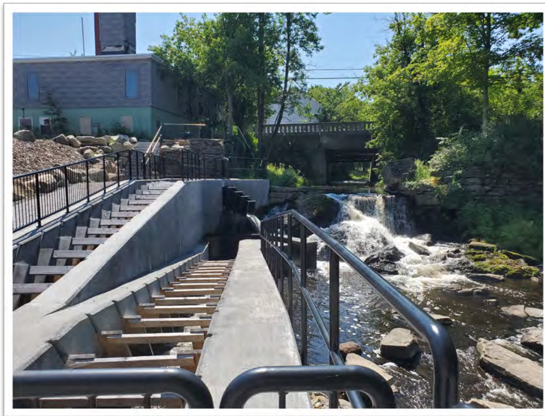
Left: After photo of engineered concrete fish ladder at Site 6.
