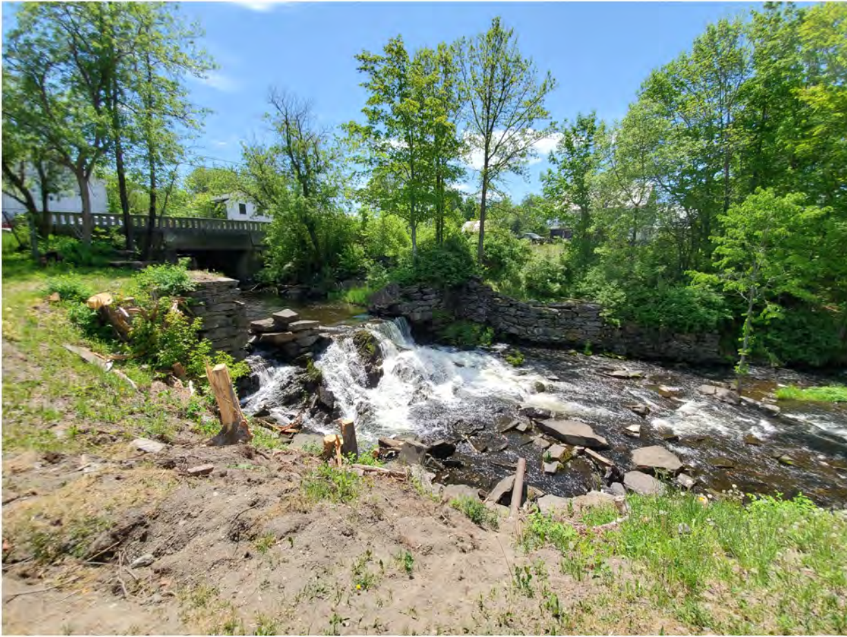
Before photo looking upstream at existing AOP barrier at Site 6.
