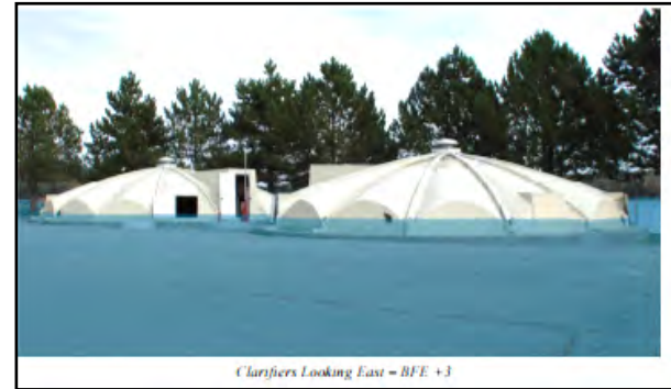
Clarifiers Looking East – BFE +3
