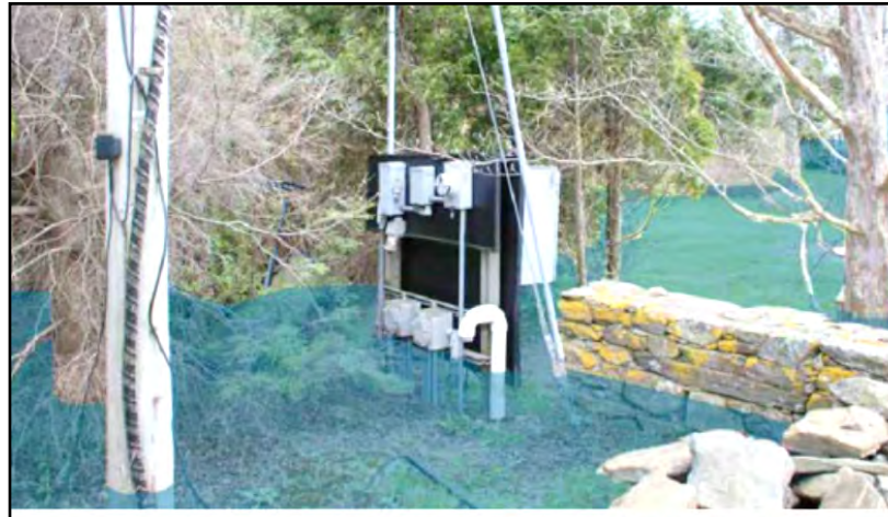
PS #12 Electrical / Controls Panel Looking South - BFE -4
