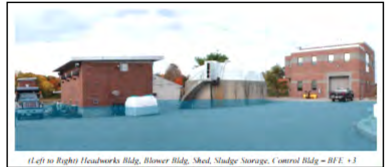
(Left to Right) Headworks Bldg, Blower Bldg, Shed, Sludge Storage, Control Bldg – BFE +3
