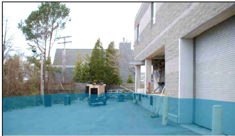
WWTP Looking West Past the Process Building - BFE -4
