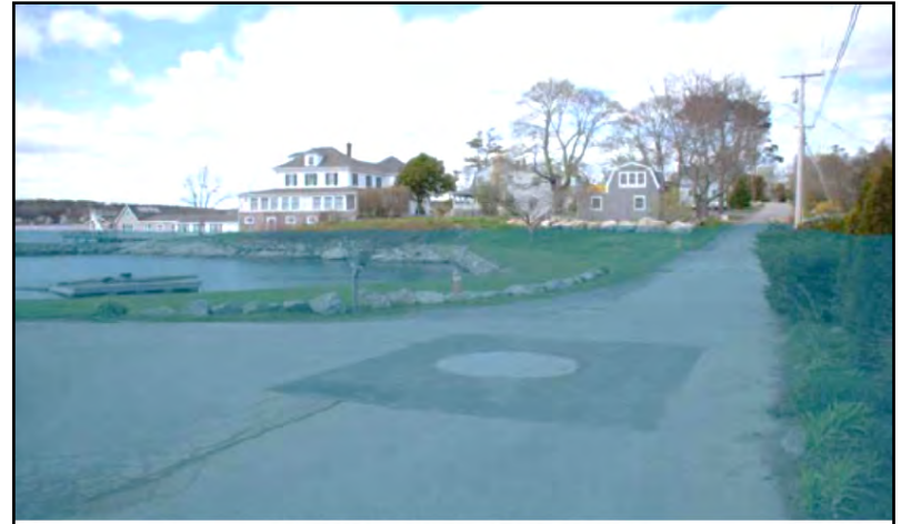
PS #12 Werwell Looking North - BFE -4
