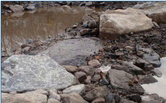
Central weir notch
