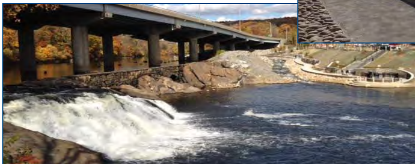
Tingue Dam (left) with Bypass NLF (above) Naugatuck River, Seymour, CT
