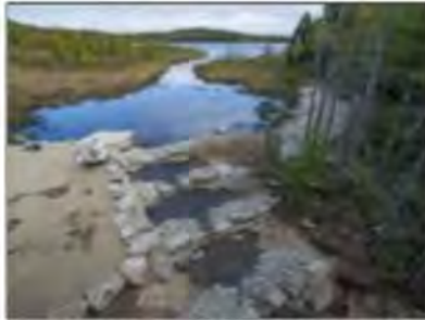
Pierce Pond, Penobscot, Maine. Engineered anadromous fish passage to Pierce Pond. Many of the thousands of ancient routes for alewives and other anadromous fish in Maine have been blocked by human activity in the form of dams, roads, unmaintained culverts and debris. The fish that annually swim up into estuaries, streams and lakes to spawn produce the trillions of young fish that return to the Gulf of Maine. They become the base of the food chain for life in the Gulf of Maine. Ken Woisard photo
