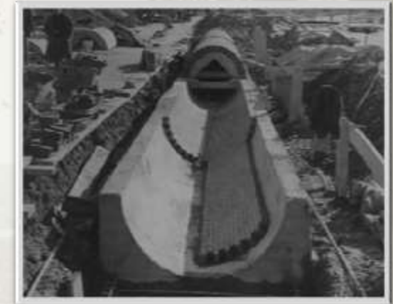
Portland West Side Interceptor, 1940
