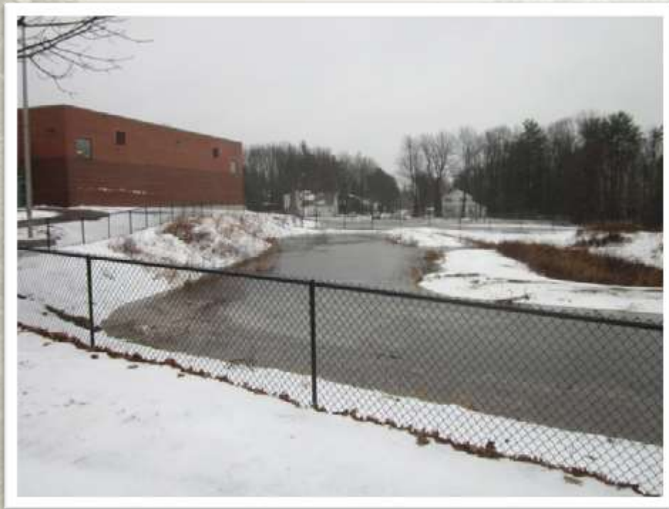
Bartley Ave to Rustic Ln Sewer Separation Project, December 2012
