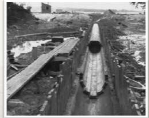
Portland Dartmouth Street Combined Sewer, 1918
