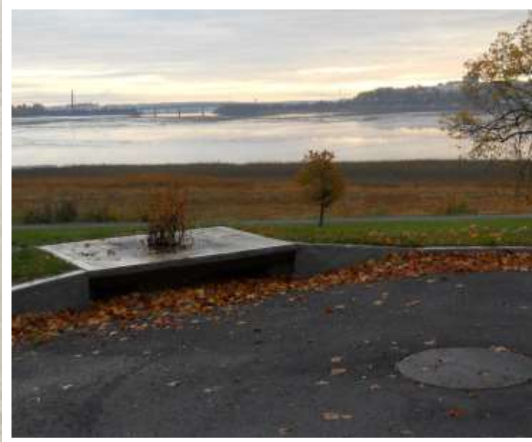
Mackworth & Austin Streets Clifton Street Sewer Separation 2009-2010
