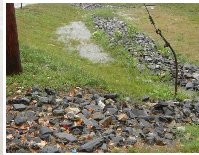
Read Street Sewer Separation 2008-2009
