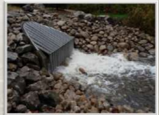
Rockland Avenue Storm Drain Outfall Rehabilitation, 2014
