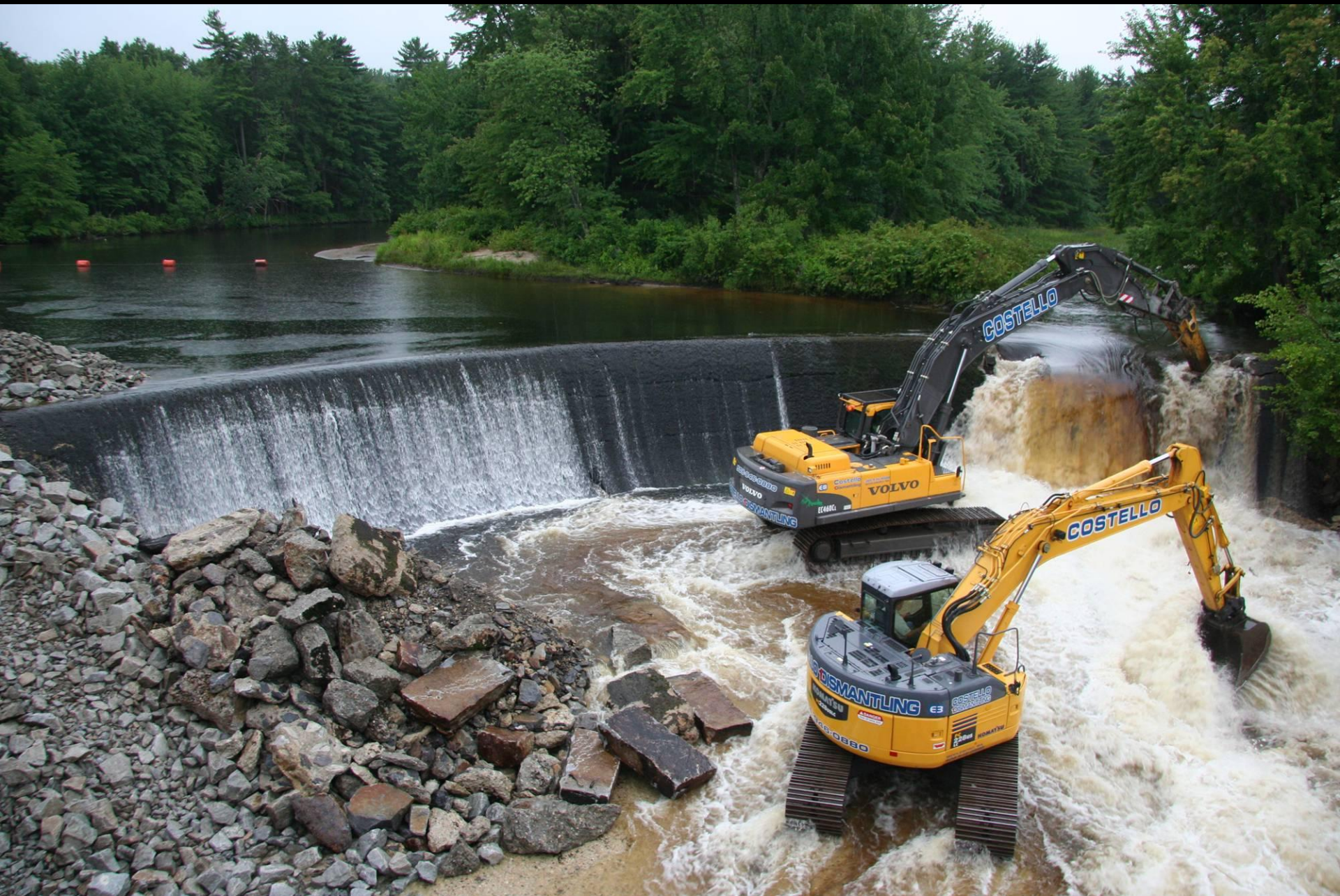
Merrimack Village Dam, Souhegan River, NH (August 6, 2008)
