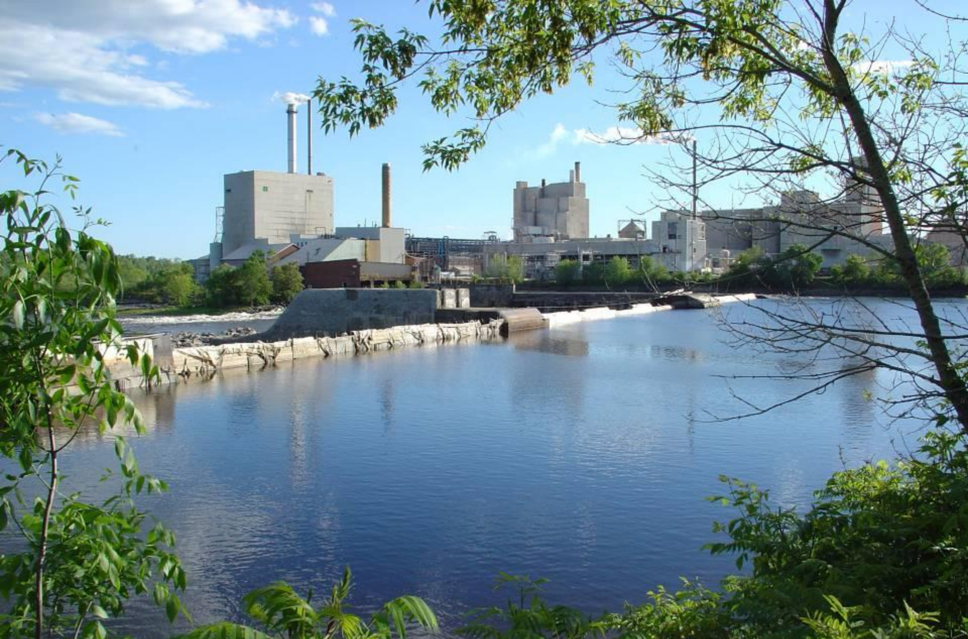
Existing Conditions Great Works Dam MMI Engineering
