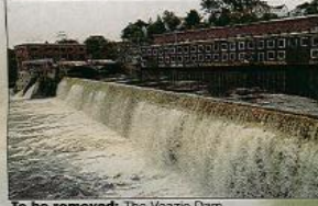
To be removed: The Veazie Dam
