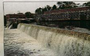
To be removed: The Veazie Dam
