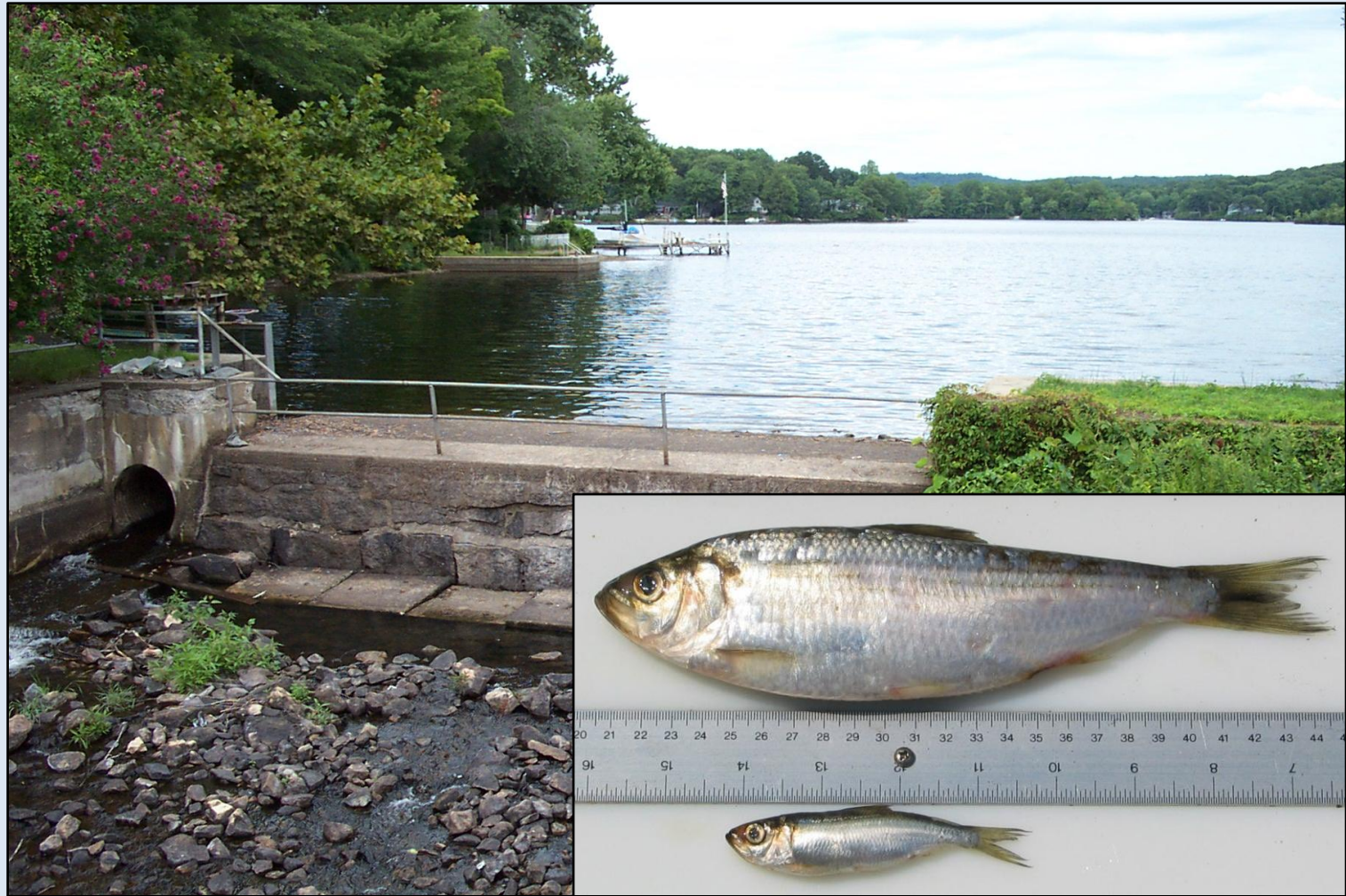
Rogers Lake Restoration Project, Old Lyme, Connecticut
