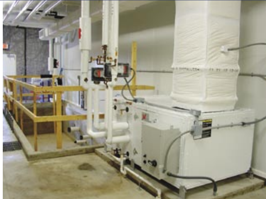
Environmental control system for the cod broodstock unit.
