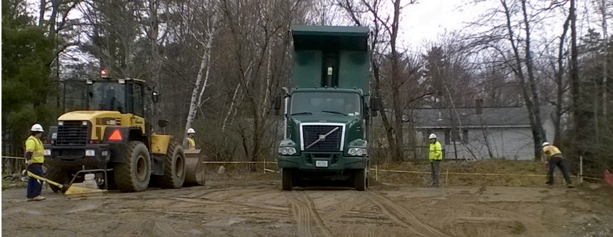
Photo 3: Placing and compacting fill
