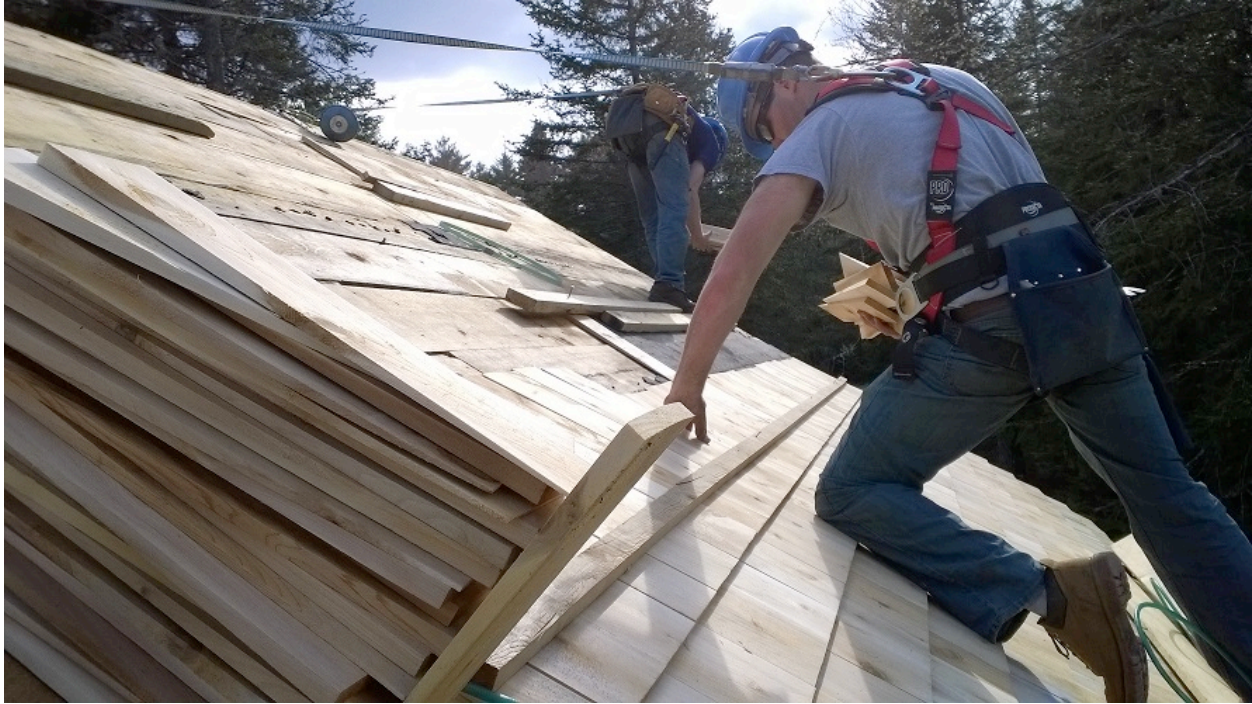
Photo 2: The crew at work with fall protection, installing new shingles
