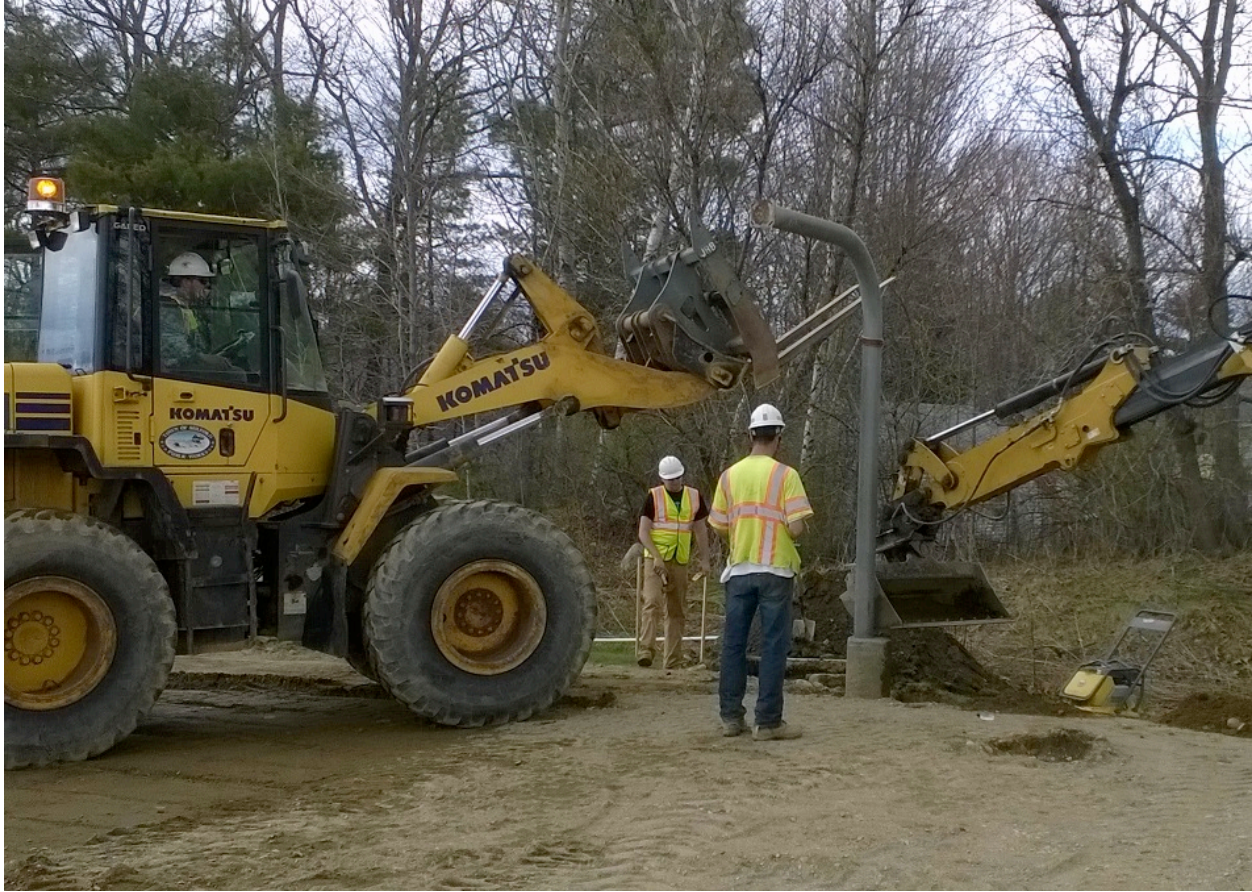
Photo 4: Setting the basketball posts
