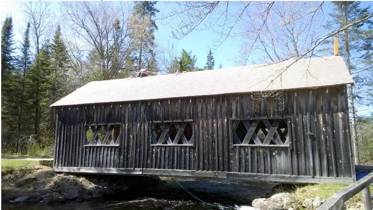
Photo 1: The covered bridge with one side finished
