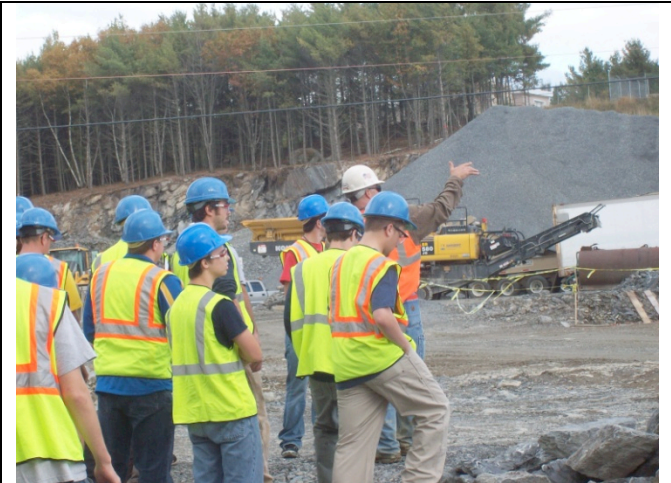
Sargent Corporation: National Guard Training Facility earthwork in Bangor
