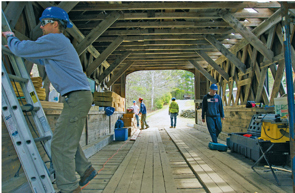
Restoration of a covered bridge.
