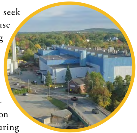
Maine-based startup GoLab is expected to start making climate-friendly wood-fiber insulation in this former Madison paper mill in 2021.
